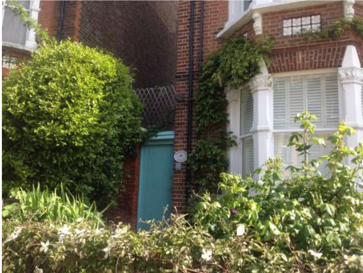
Image 1 – Pedestrian access point. No heavy machinery can or will be brought on site.
