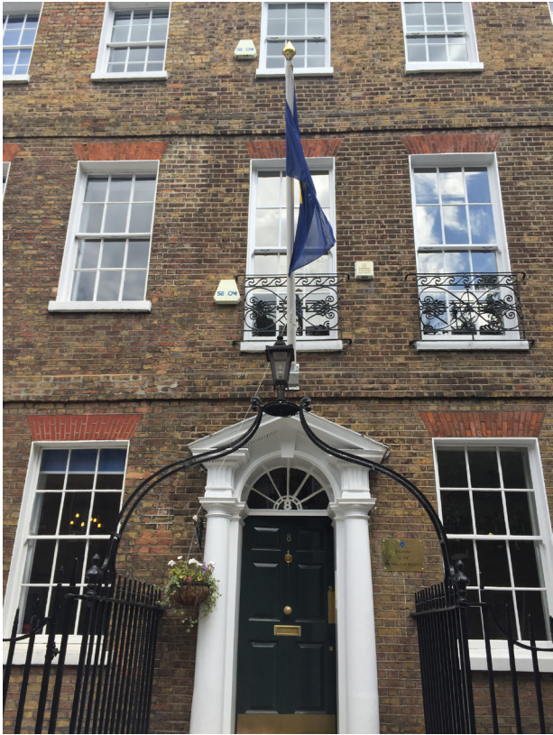
Existing front facade
