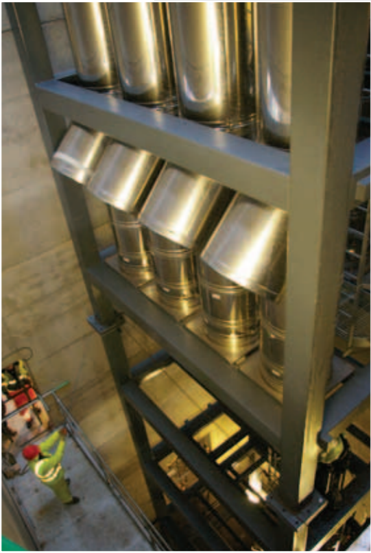
Chimneys ready to be connected to the appliances
