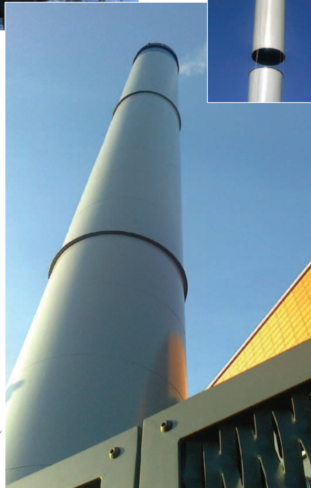
Completed 40m multicore chimney
