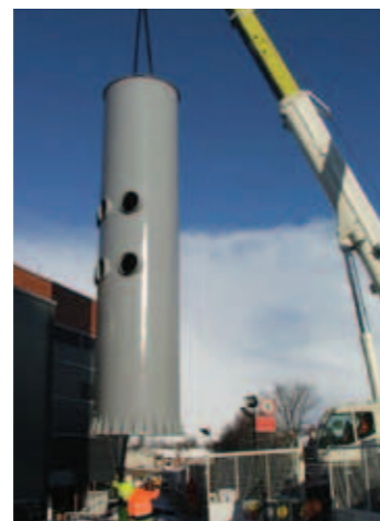
Base section goes into place
