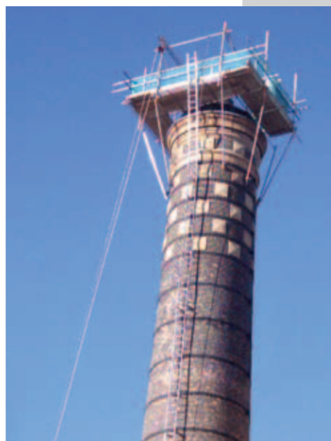
Chimney relining in progress
