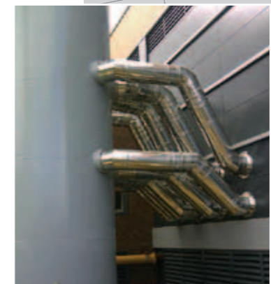
Connections to the appliance in the energy centre
