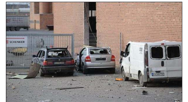
The impact of Friday's massive blast damaged cars parked near the site
