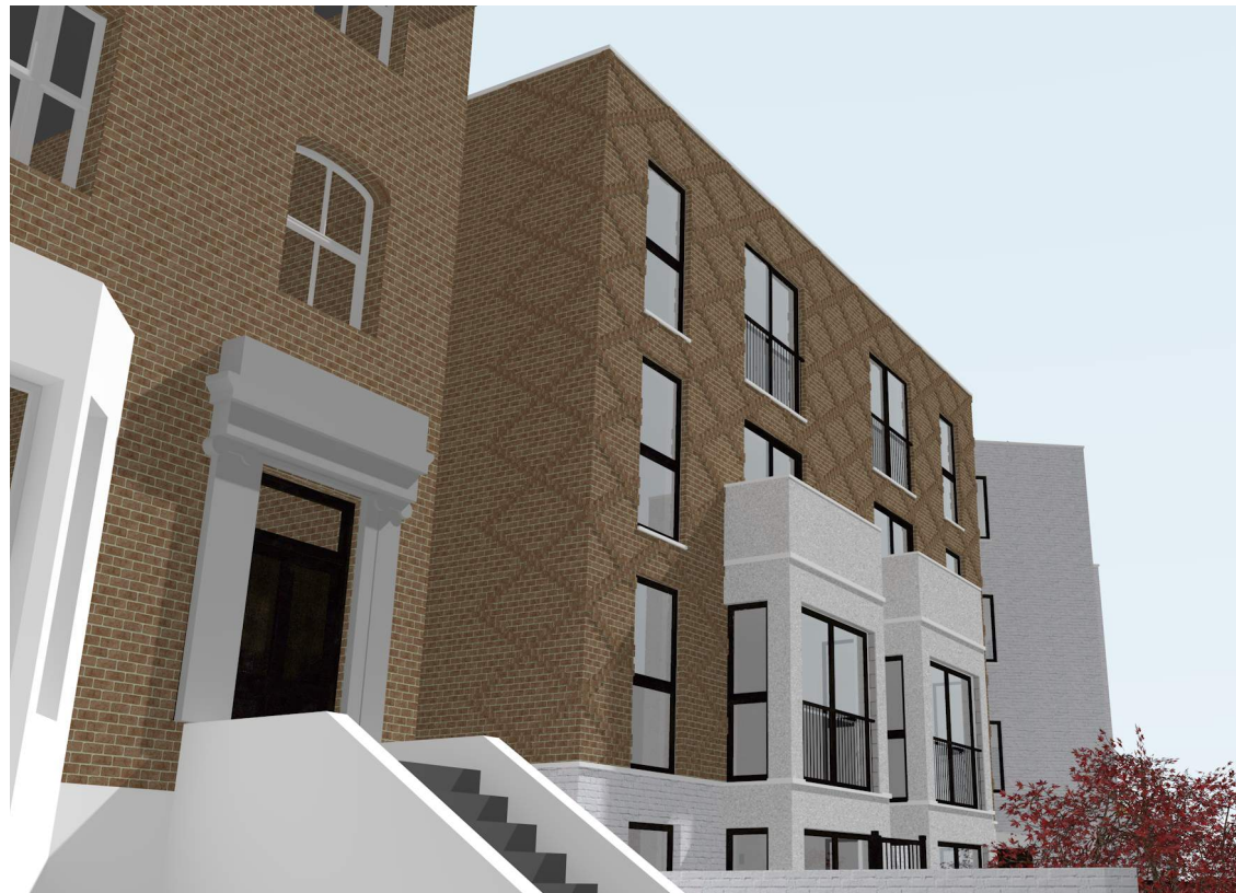
Projecting relief pattern continues around corner
