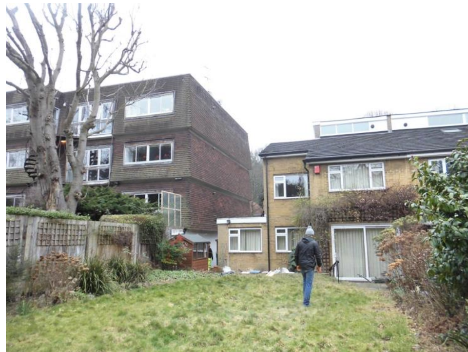
Photograph 6 – Rear Elevation of Property
