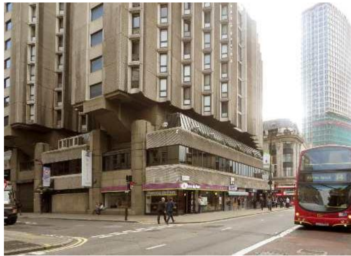
View of the Hotel from southern approach
