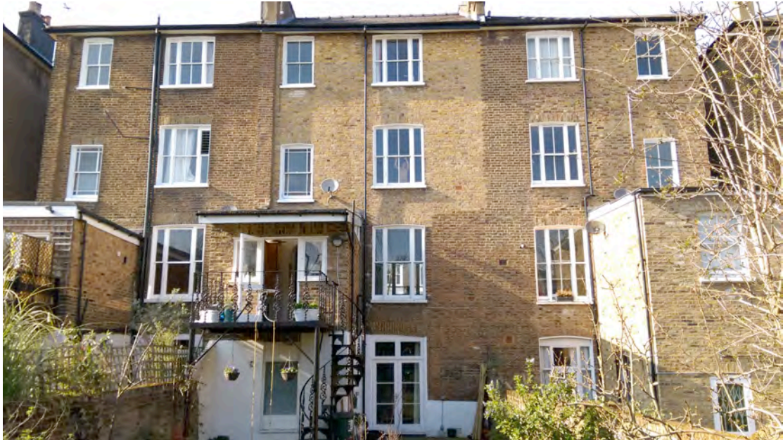
existing rear elevation showing existing 2-storey extension
