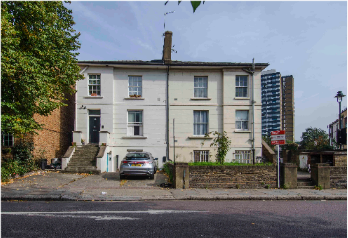
58 St Pancras Way London NW1 9NB Front Elevation (West)
