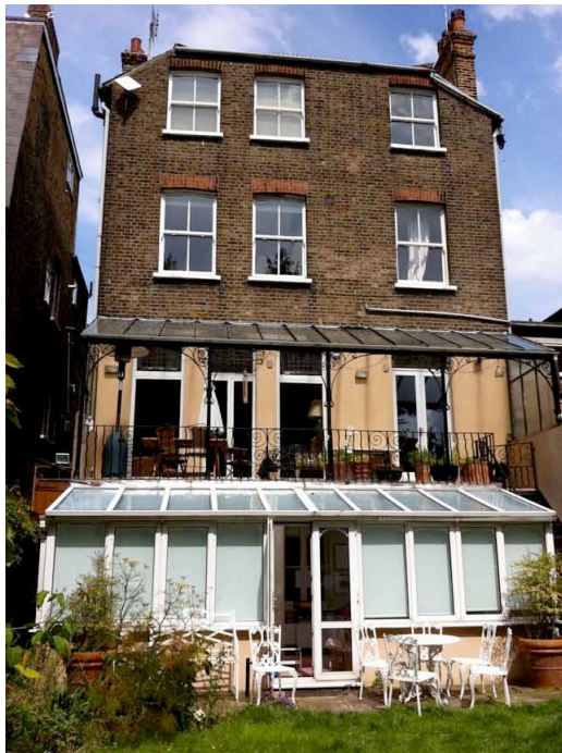
Rear elevation showing existing extension
