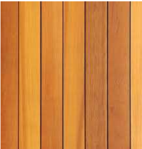
Figure 4; Cedar cladding, this will turn to a silver grey colour
