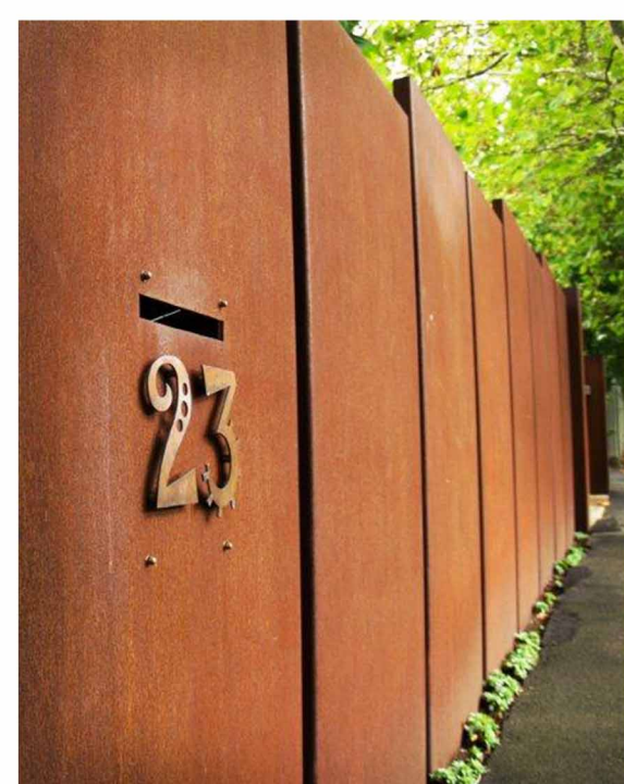
Cor-ten Steel Palisade
