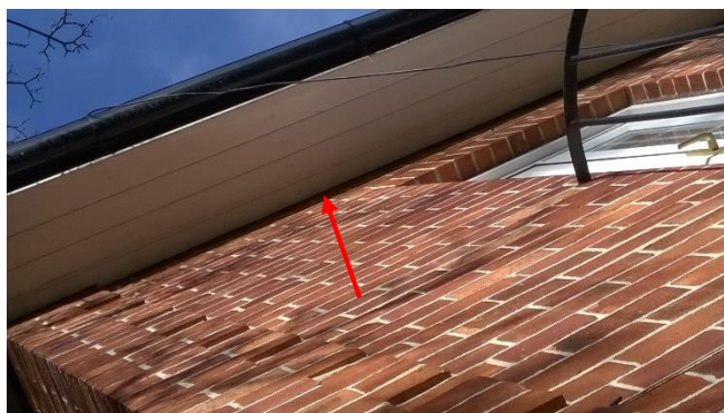
Plate 4.3: Gap between soffit and brickwork.
