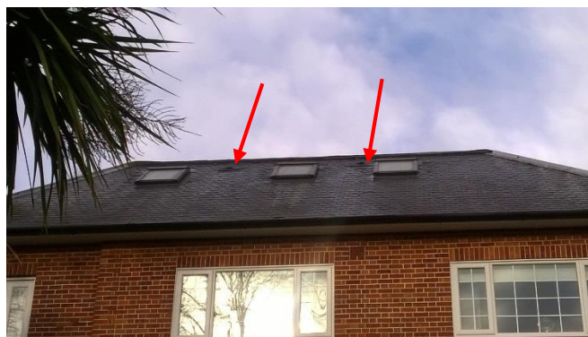
Plate 4.3: Missing and slipped tiles of southern elevation.
