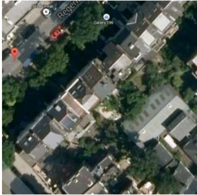
Satellite image showing opposite terrace block showing the presence of various roof lights and roof extensions to the roof slopes
