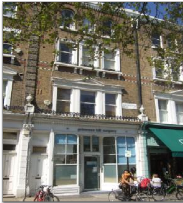
Above: View of front elevation of 99 Regents Park Road
