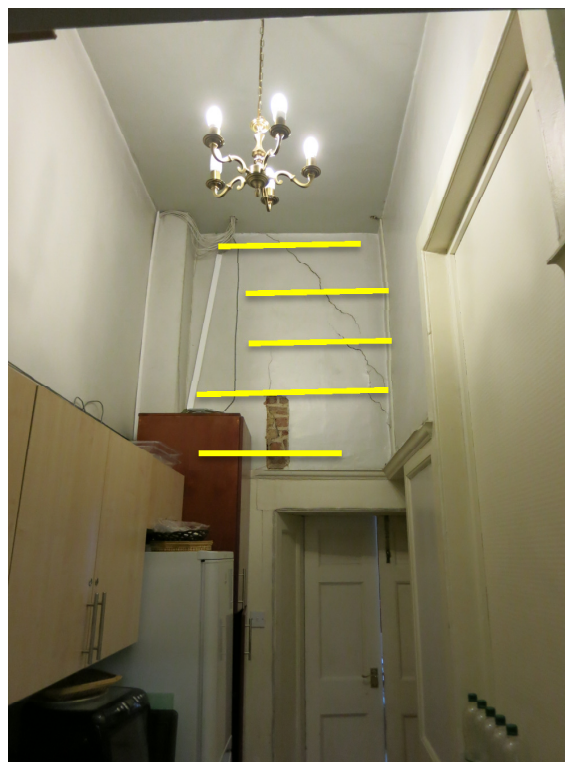
02 Eastern end of first floor corridor
