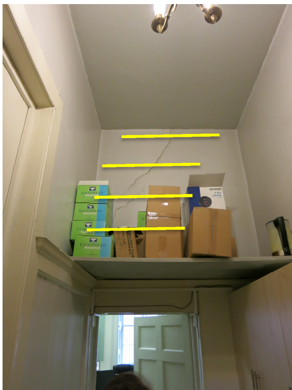
01 Western end of first floor corridor
