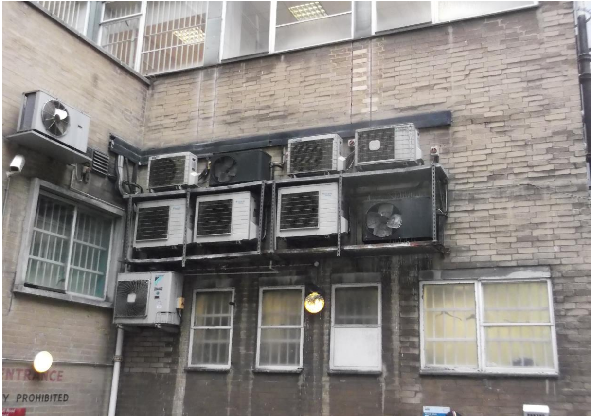
View of the 9no. units plus the window to be adapted.
