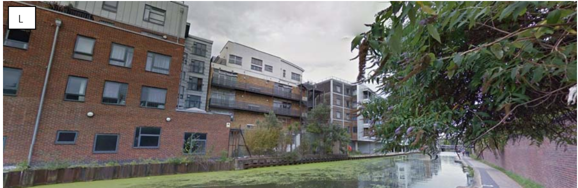
Image L: View from public footpath of site and frontage onto the canal
