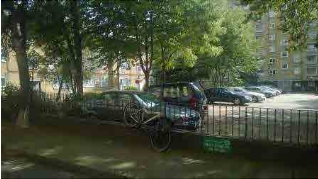
Image 1: Plot 1 - car park and landscaped area from the west.
