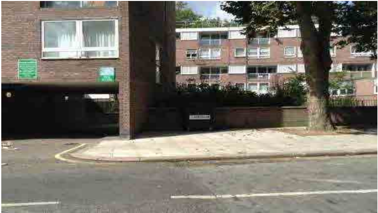
Image 10: Plot 5 - access to the underground parking for Rothay Block.
