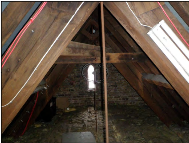
Photograph 3: St. Bede's Hall within the elevated tower section to the south of the building.
