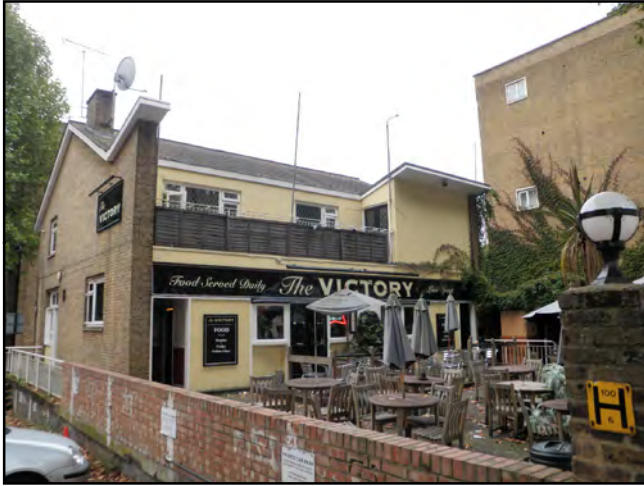
Photograph 1: The Victory Public House is a functional public house assessed as having low potential to support roosting bats.
