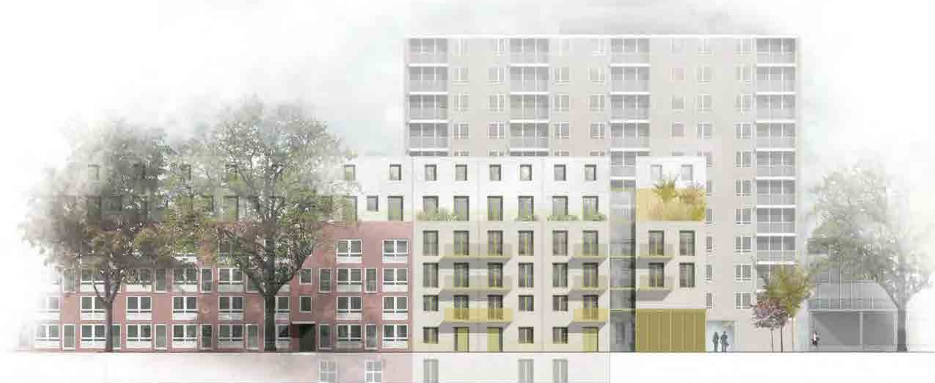
Principal Elevation along Albany Street
