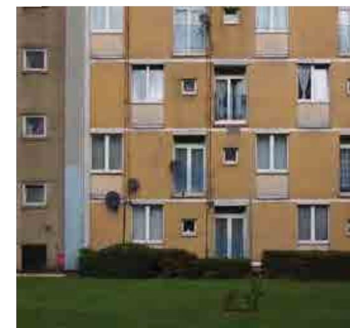
Apartment buildings are often directly adjacent to well-kept public landscape affording open aspect and generous shared gardens
