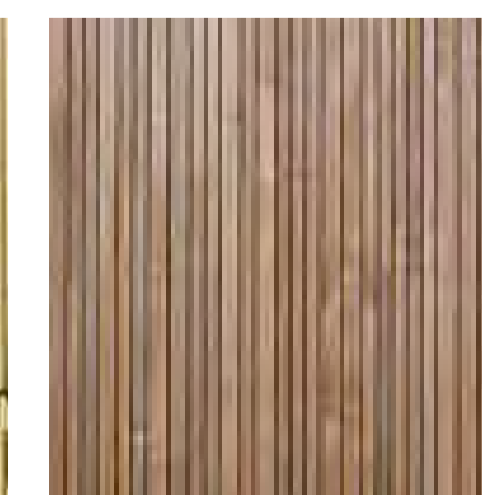
Timber cladding - Balcony
