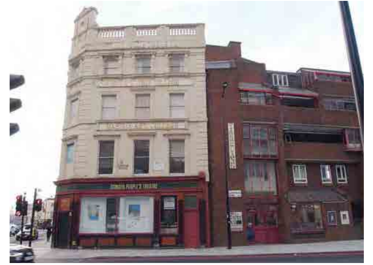
The existing CPT building has its access to the upper floors via the neighbouring building
