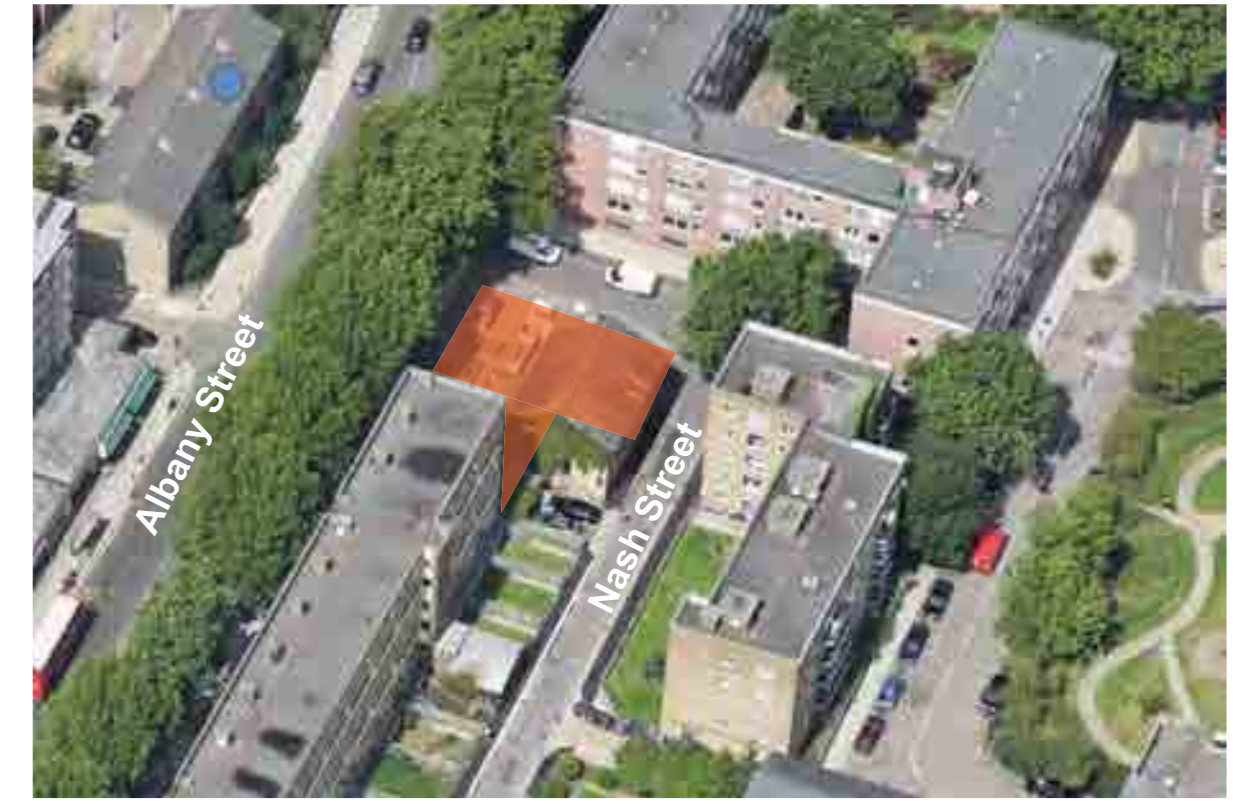
Aerial view of the existing site
