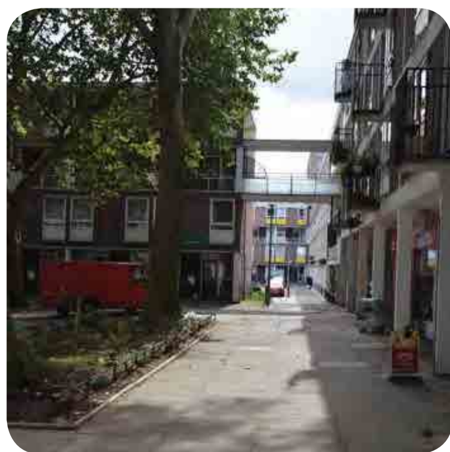
Level changes and a fractured street pattern make navigation difficult around the area.
