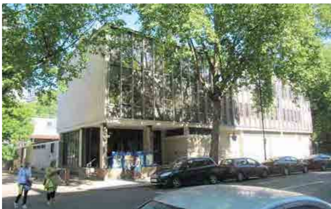
Existing: the former police station building
