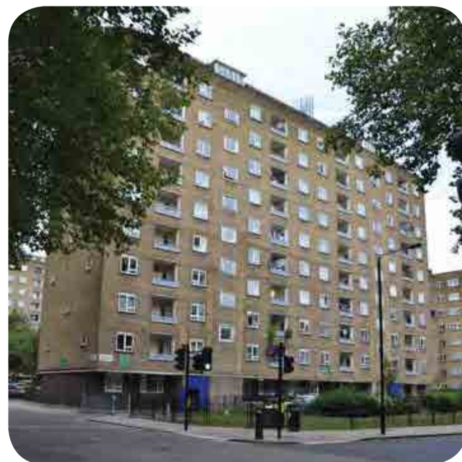
Parking needs organising to improve the public realm.
