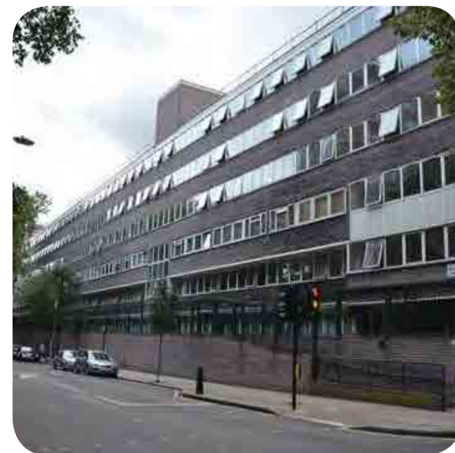
Surrounding buildings don't have a good relationship with the street and public realm.
