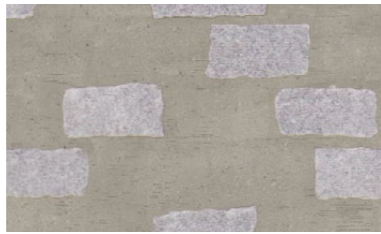
2. Granite setts within concrete path surface
