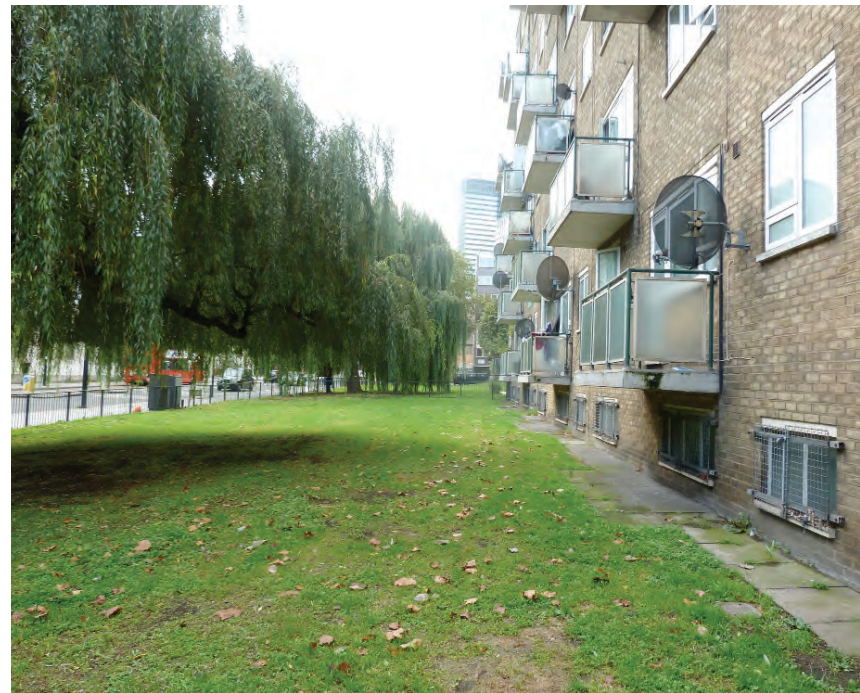
Existing amenity space to The Tarns with projecting balconies overlooking Hampstead Road
