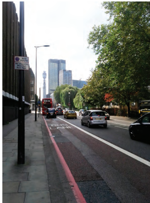
Green edge to estate on Hampstead Road defined by willow trees on the Former One Stop Shop plot and The Tarns
