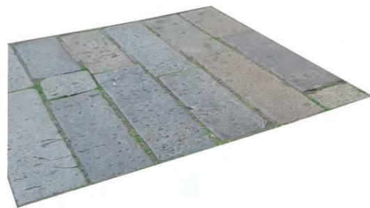
Reclaimed granite kerb mats to existing residential entrances
