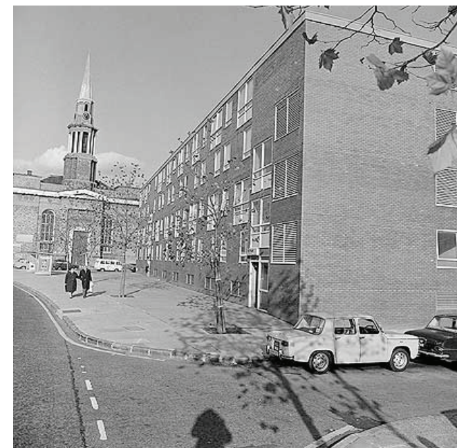
The Civic space facing Rothay and St. Georges' Cathedral during the 50s
