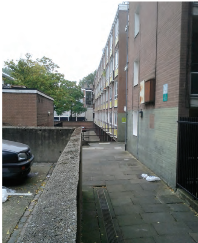
A mix of climbing plants are proposed to the west-facing wall of Clarence Gardens with yellow flowers
