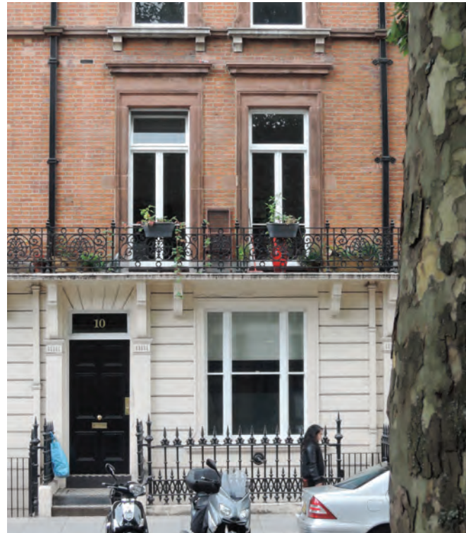
Colosseum Terrace: its elevations have a distinct hierarchy and are decorated with stucco, brick and stone details and metal filigree.
