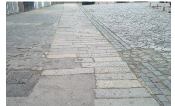
5. Existing granite cobbles
