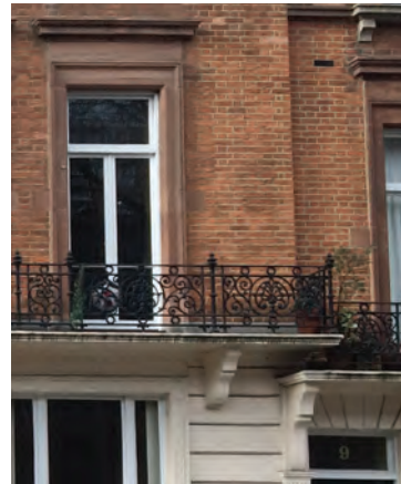
1 Stucco to mark the base of the building, metalwork and stone details on Colosseum Terrace
