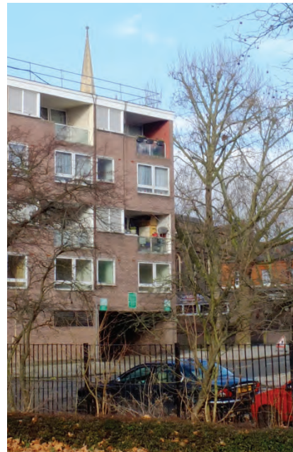
Existing punched balconies to Rothay
