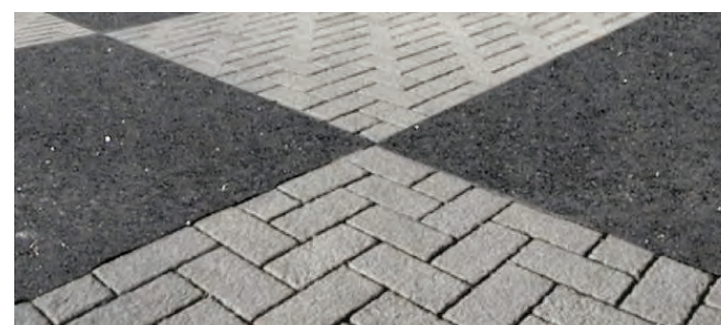
3. Asphalt and granite setts chequerboard
