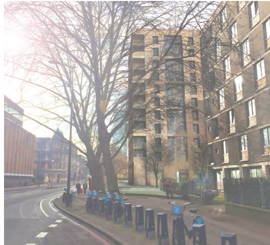
View 1 Hampstead Road looking South, with the proposed Newlands plot beyond Cartmel
