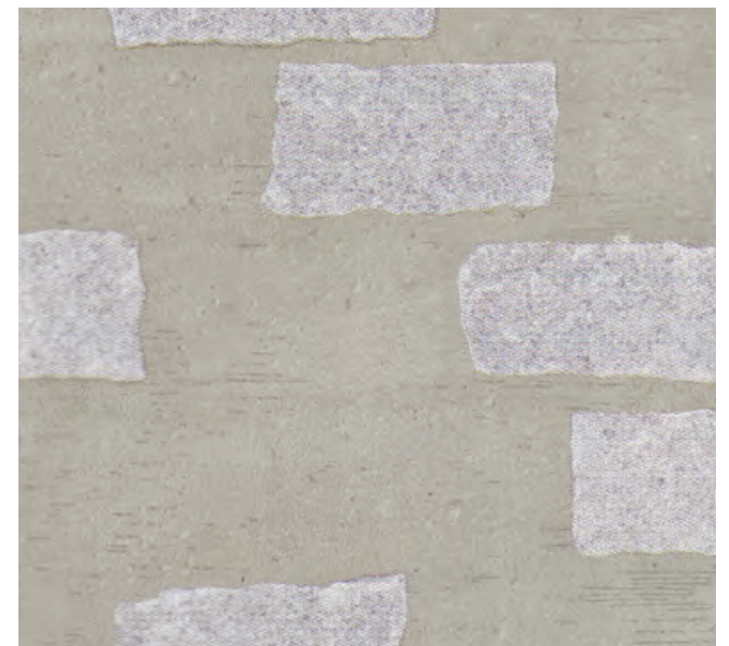
6. Granite setts within concrete path surface
