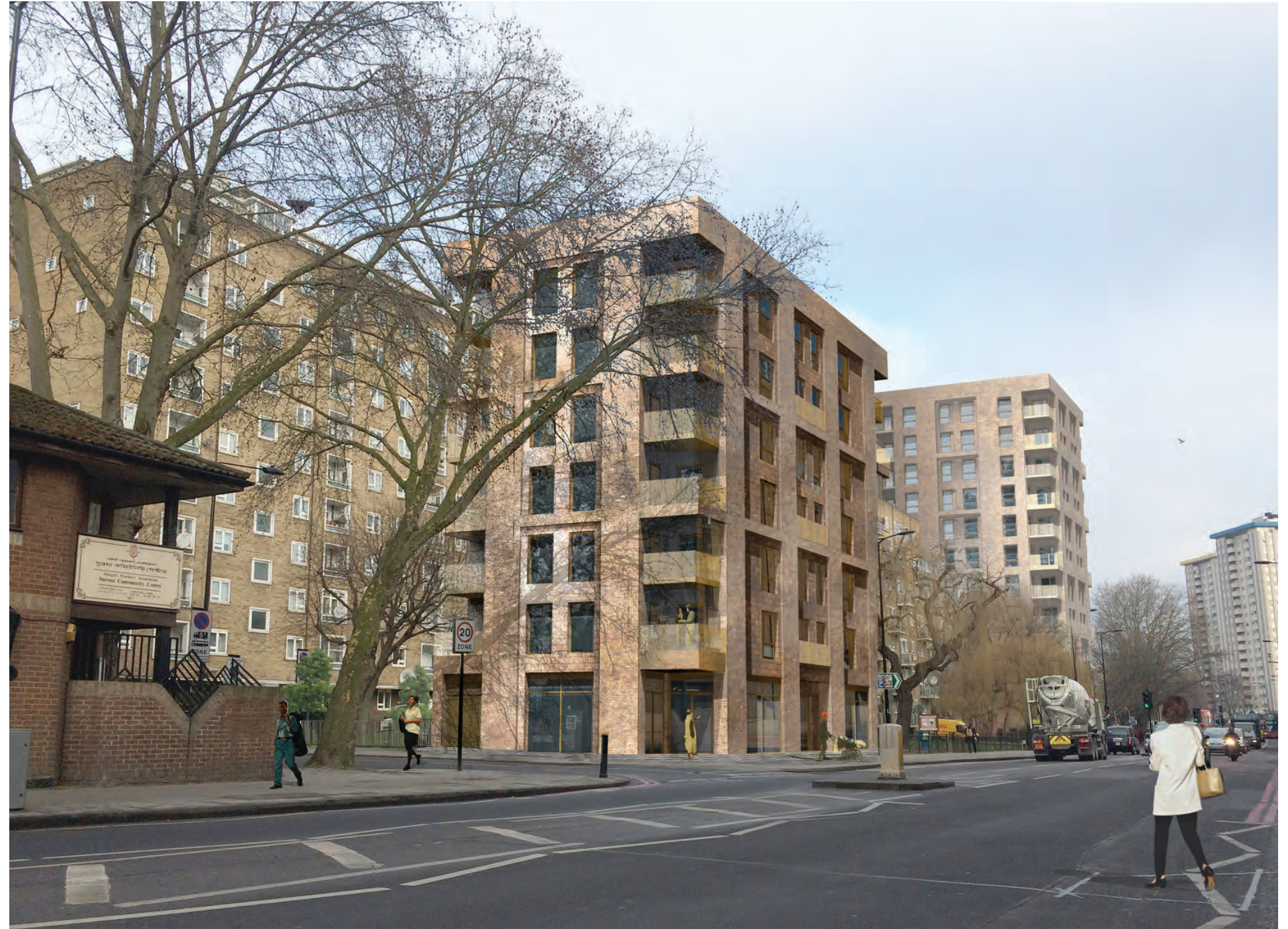
View of the corner of Robert Street and Hampstead Road
