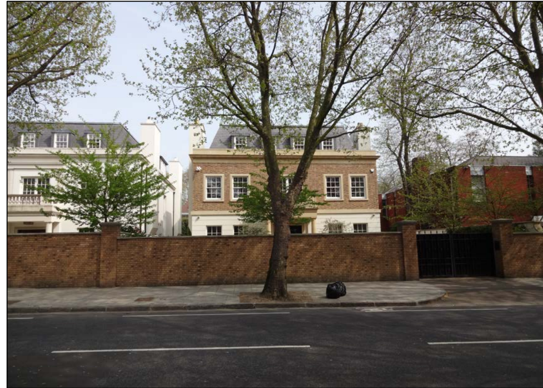
PHOTO B (Existing front elevation from Avenue Road)
