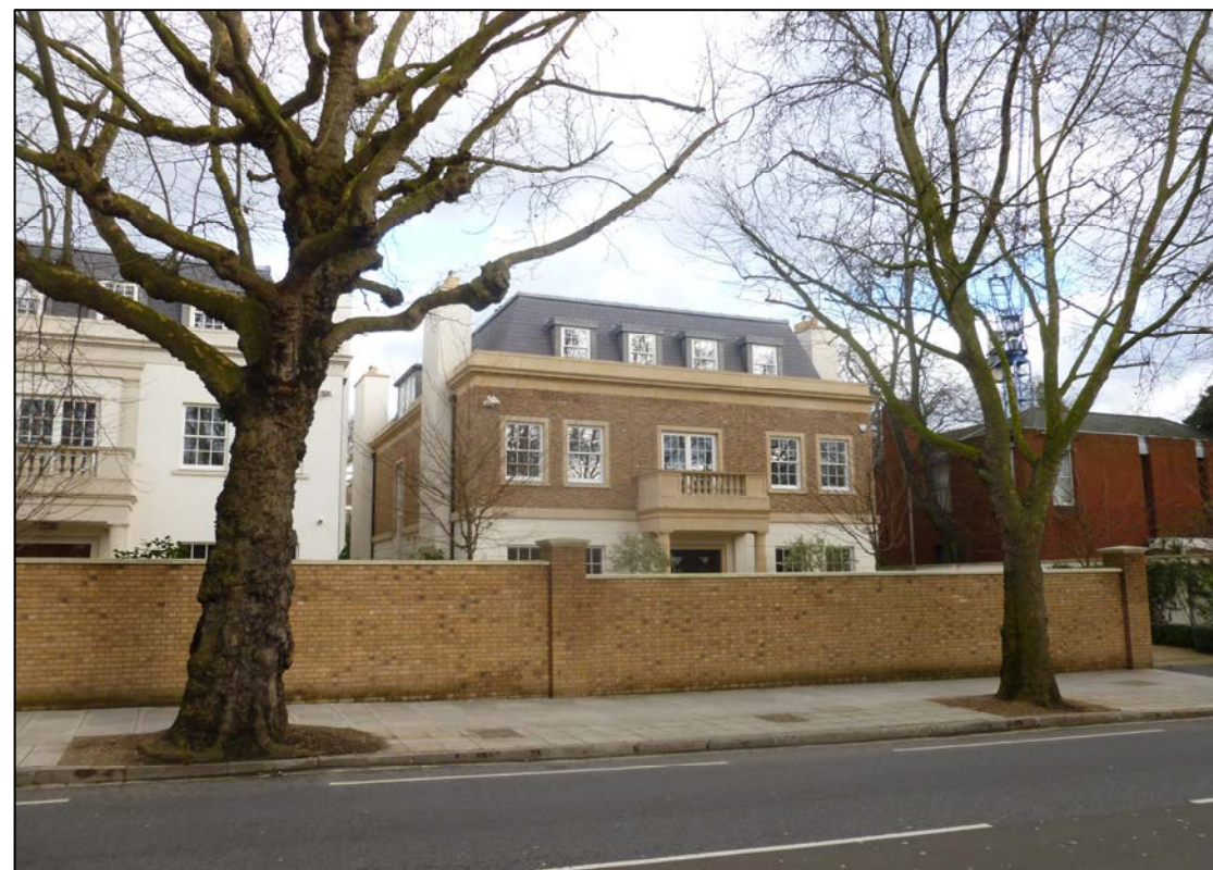
PHOTO D (Existing front elevation- viewed from North)
