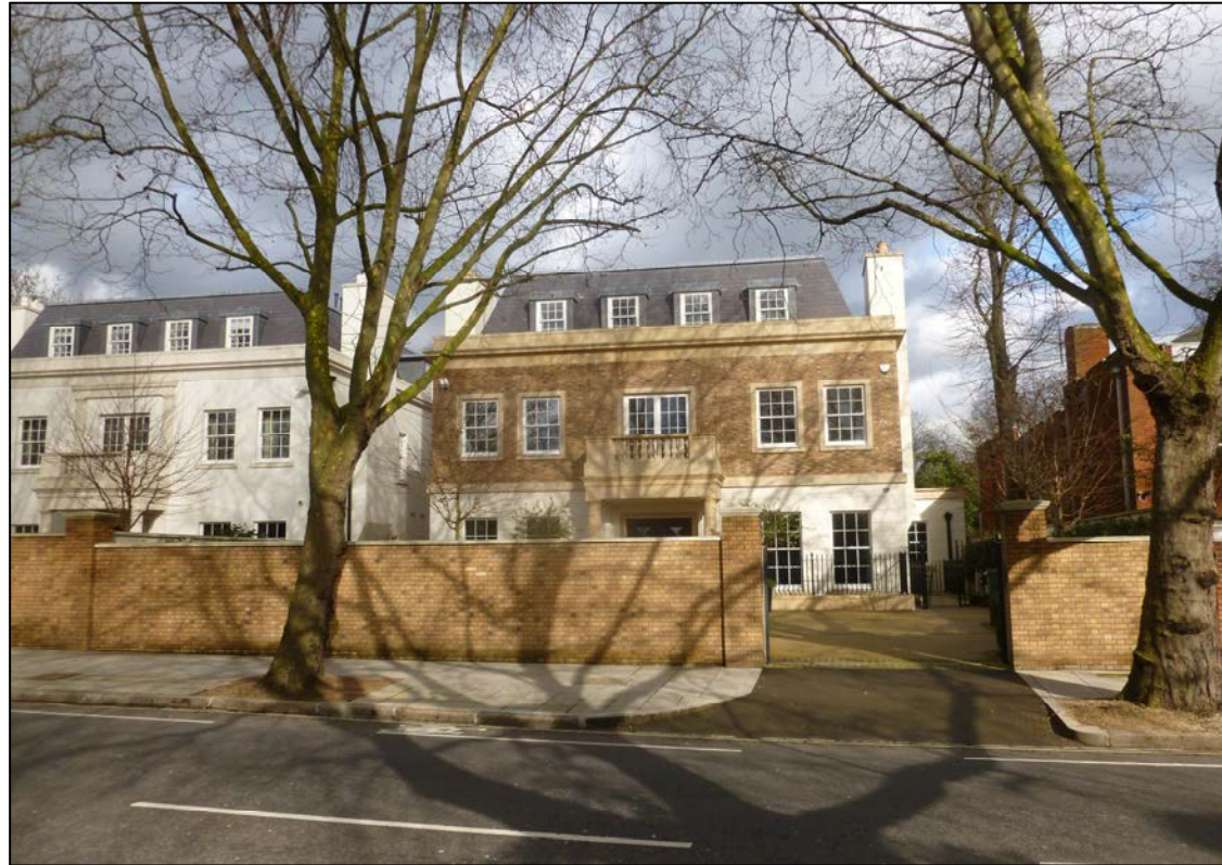
PHOTO A (Existing entrance and front elevation)
