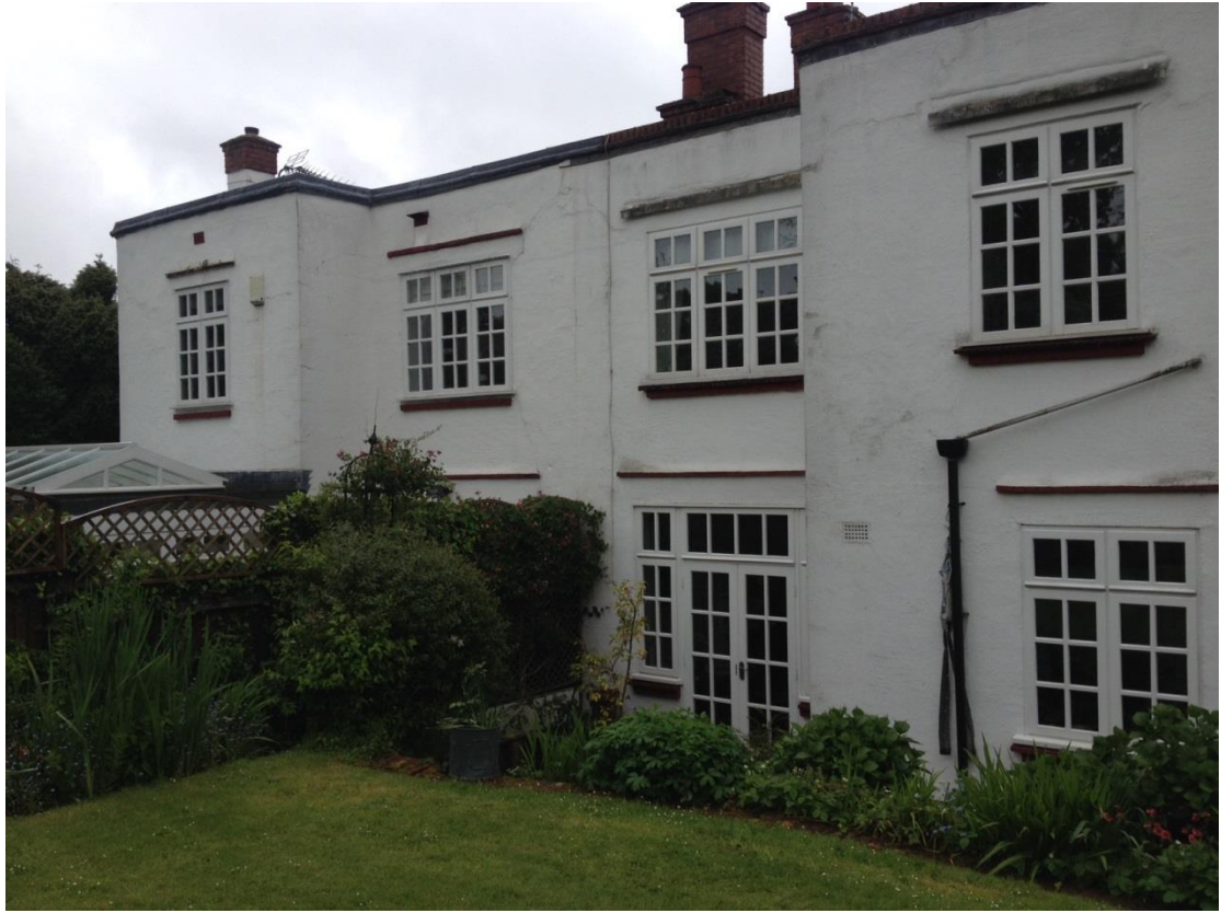
Photo 3- Rear elevation from 31 Makepeace Avenue
