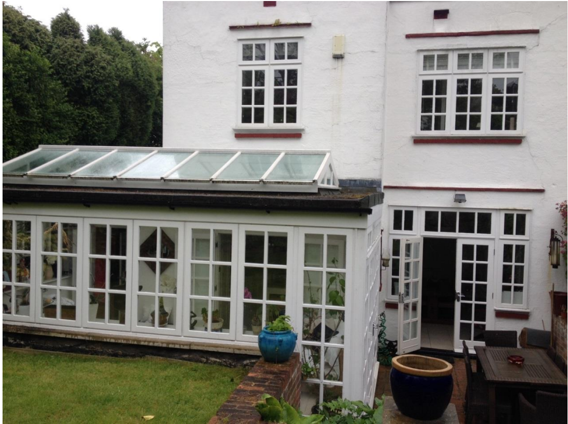
Photo 1- Existing rear elevation and rear extension on left hand side
