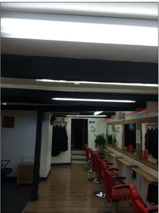
HAIR STUDIO 2 WHITE PLASTIC CABLE TRUNKING TO BE ATTACHED TO THE WALL BENEATH THE TIMBER BEAMS USING LIMITED FIXINGS. NO TIMBERS WILL BE CUT OR HARMED. PROPOSED NEW TRUNKING.
