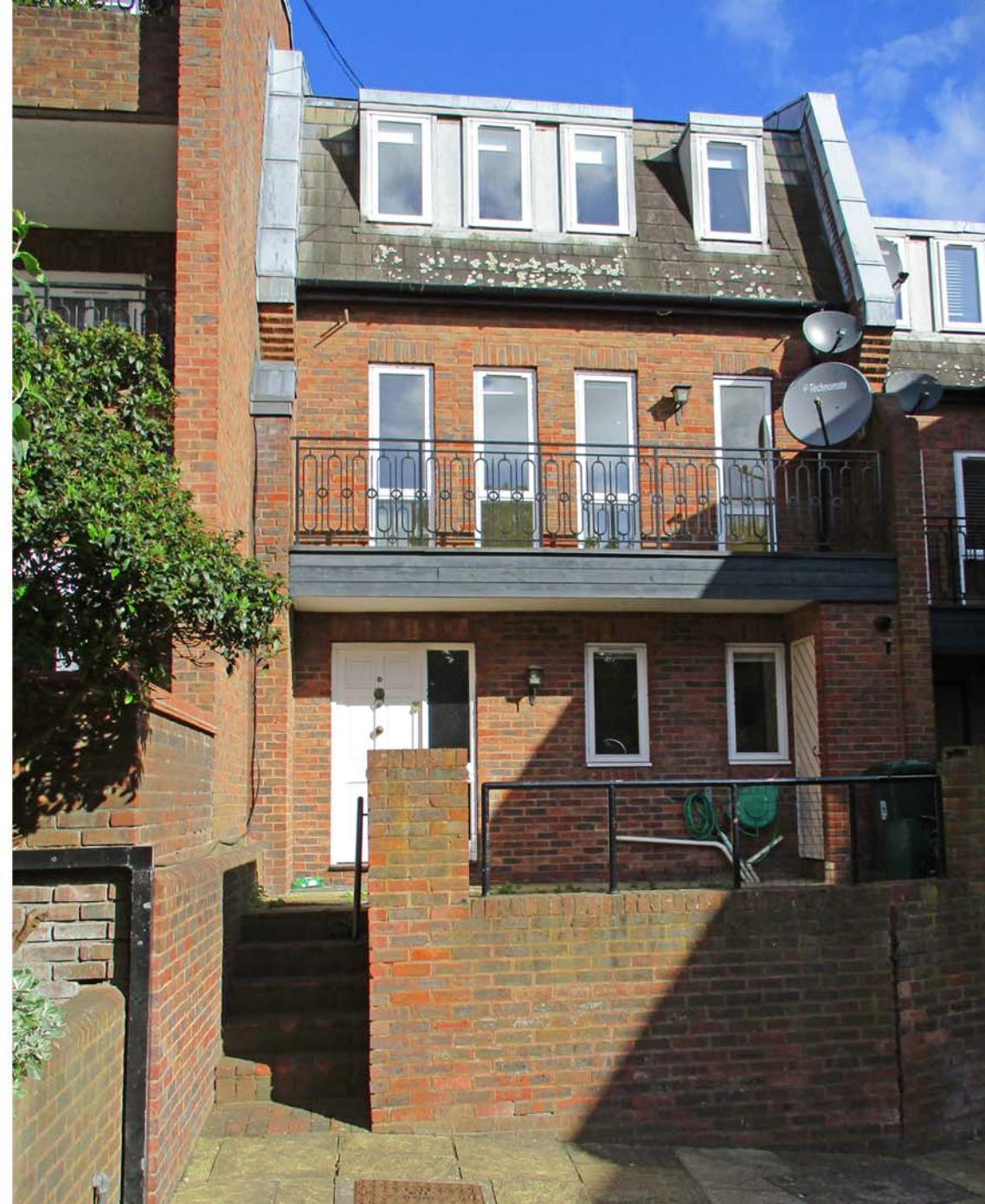
site photo : front elevation
