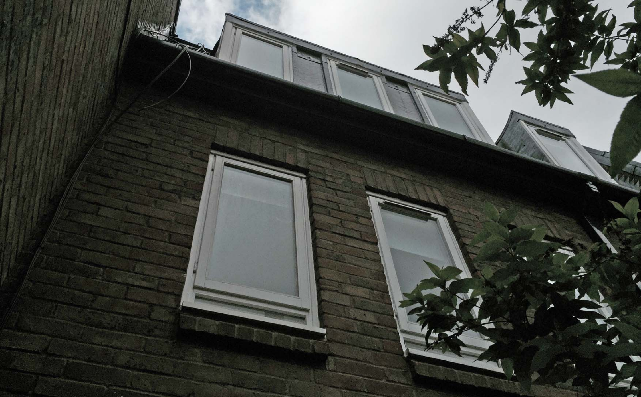
site photo : rear elevation
