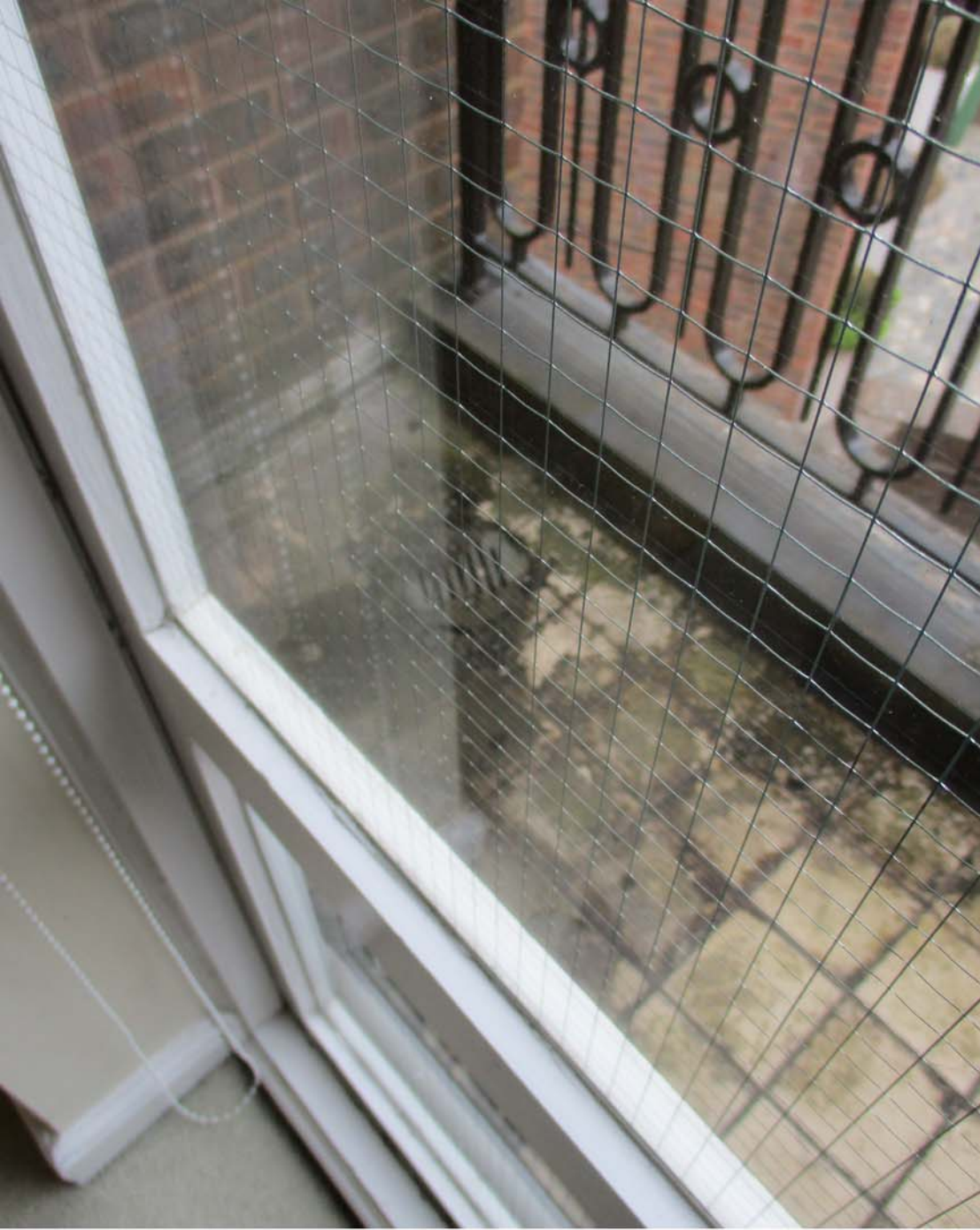
site photos : master bedroom : first floor front : note georgian wired glass side hung window + double glazed side hung windows with fixed lower pane
