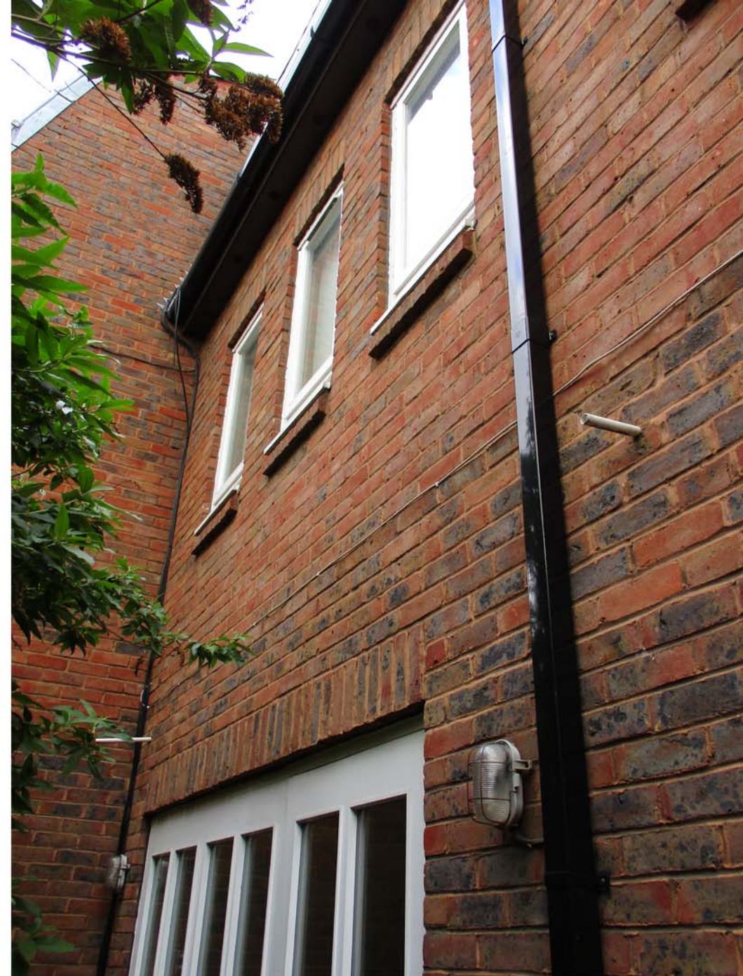
site photo : rear elevation
