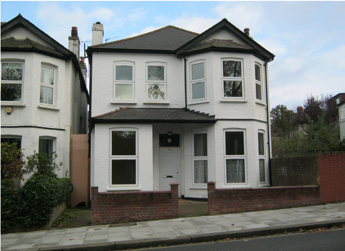
Street view of 44 Westbere Road
