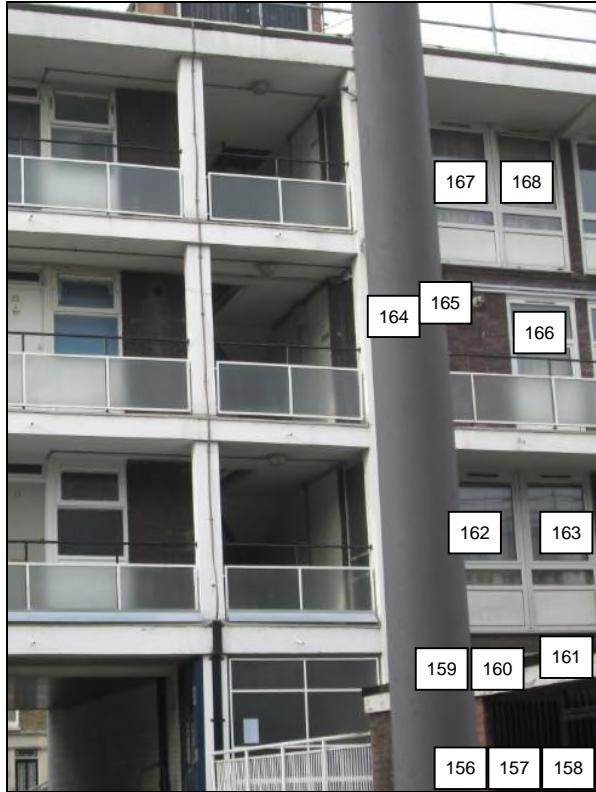
1 to 95 Troutbeck Building
