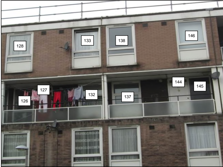
1 to 95 Troutbeck Building
