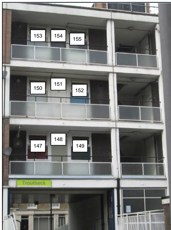
1 to 95 Troutbeck Building
