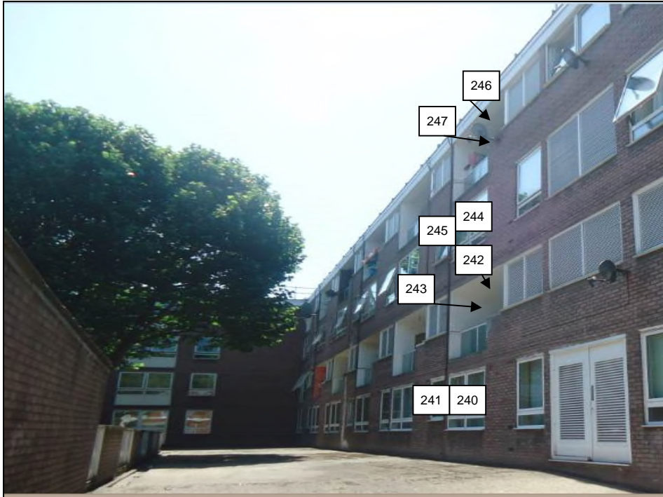
1 to 50 Rothay Red Hill Street
