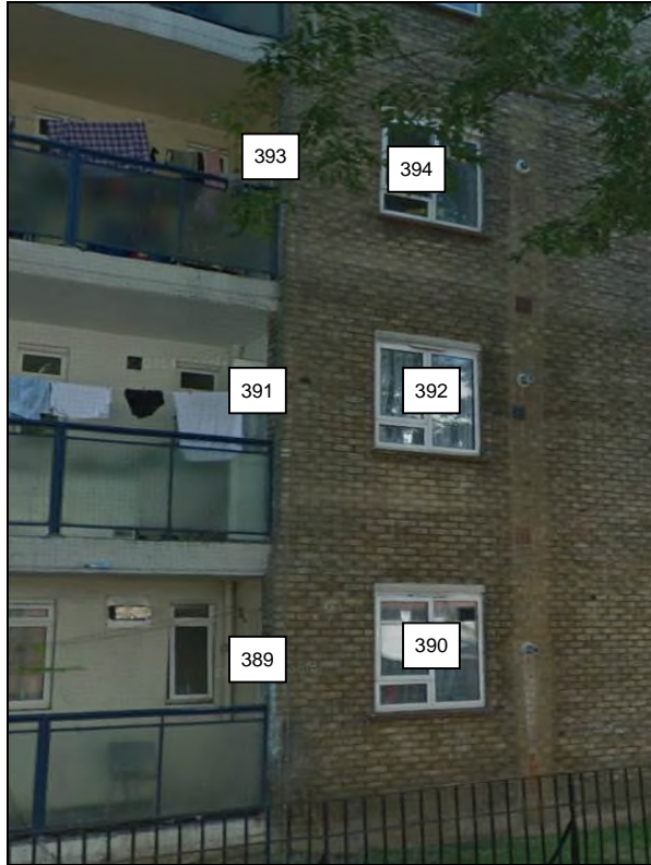
1 to 16 Ennerdale House
