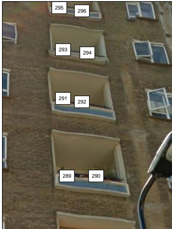
1 to 16 Ennerdale House
