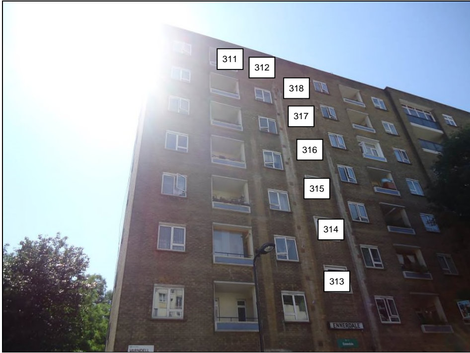
1 to 16 Ennerdale House
