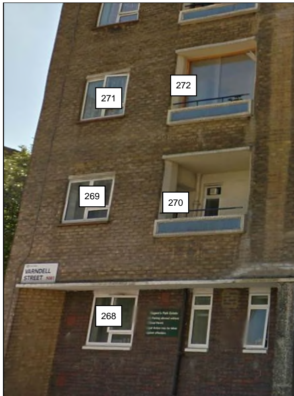
1 to 16 Ennerdale House
