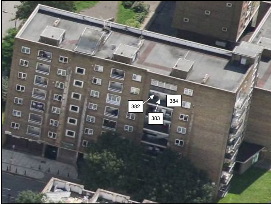
1 to 16 Ennerdale House
