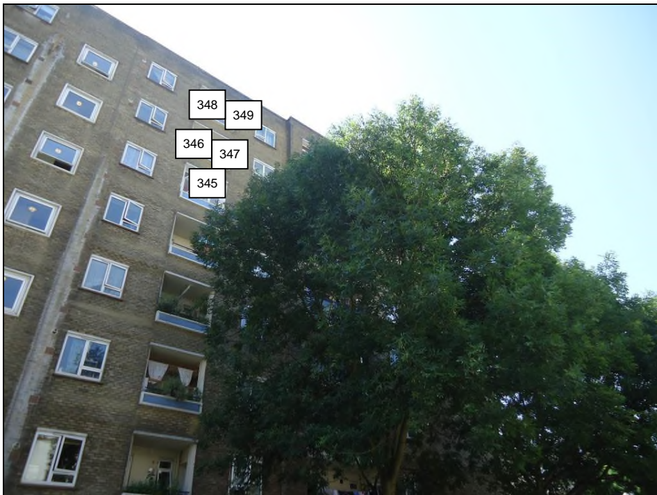
1 to 16 Ennerdale House
