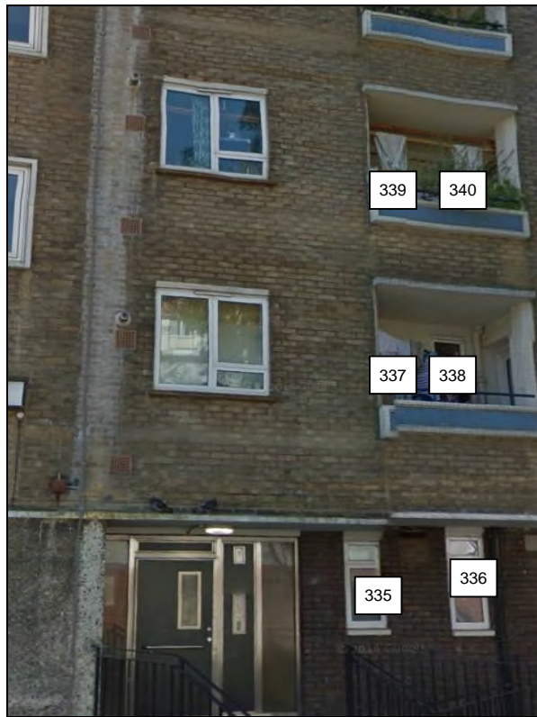
1 to 16 Ennerdale House
