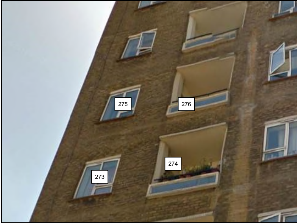
1 to 16 Ennerdale House
