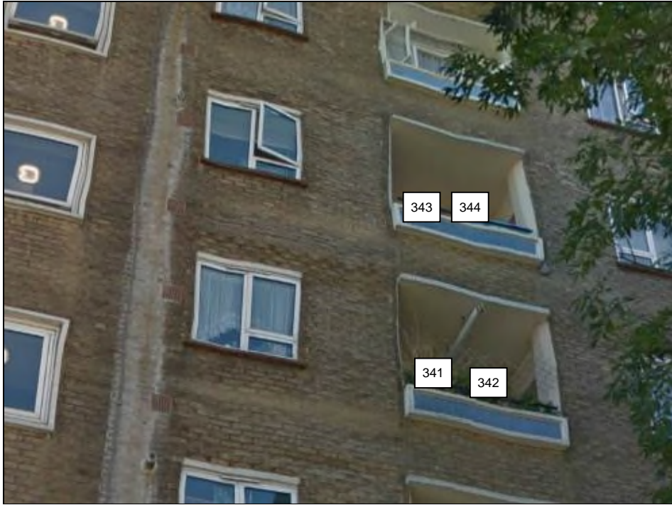
1 to 16 Ennerdale House
