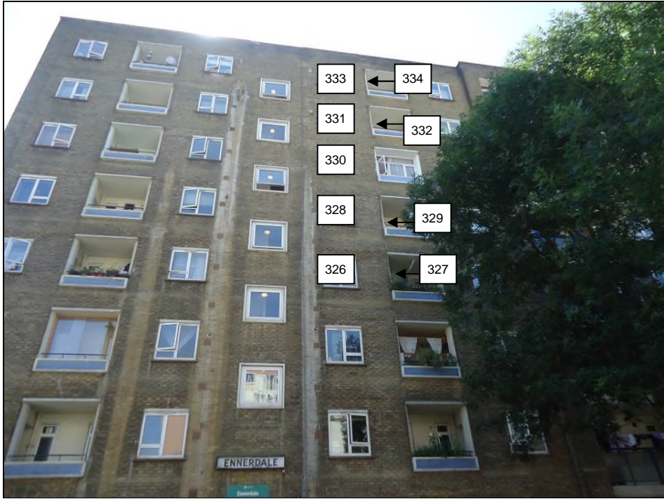
1 to 16 Ennerdale House
