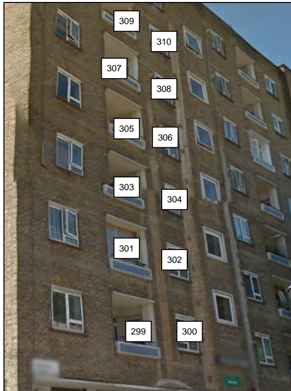
1 to 16 Ennerdale House
