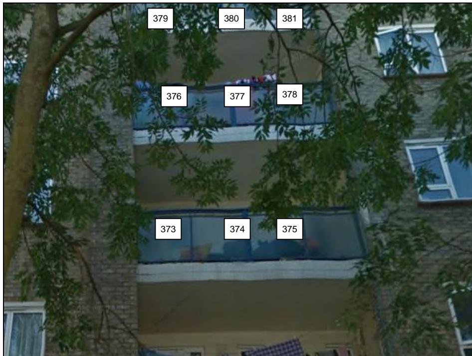
1 to 16 Ennerdale House
