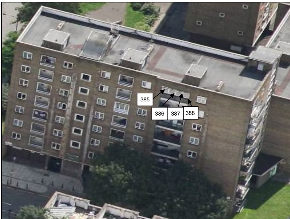
1 to 16 Ennerdale House
