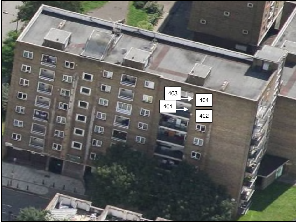
1 to 16 Ennerdale House
