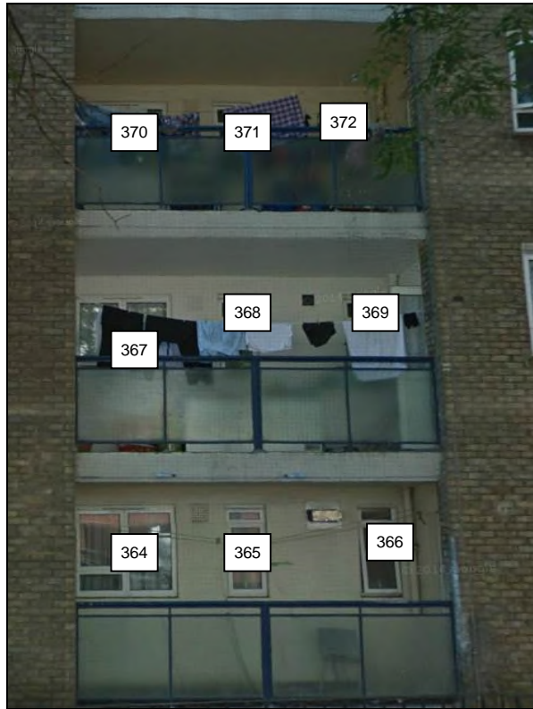
1 to 16 Ennerdale House
