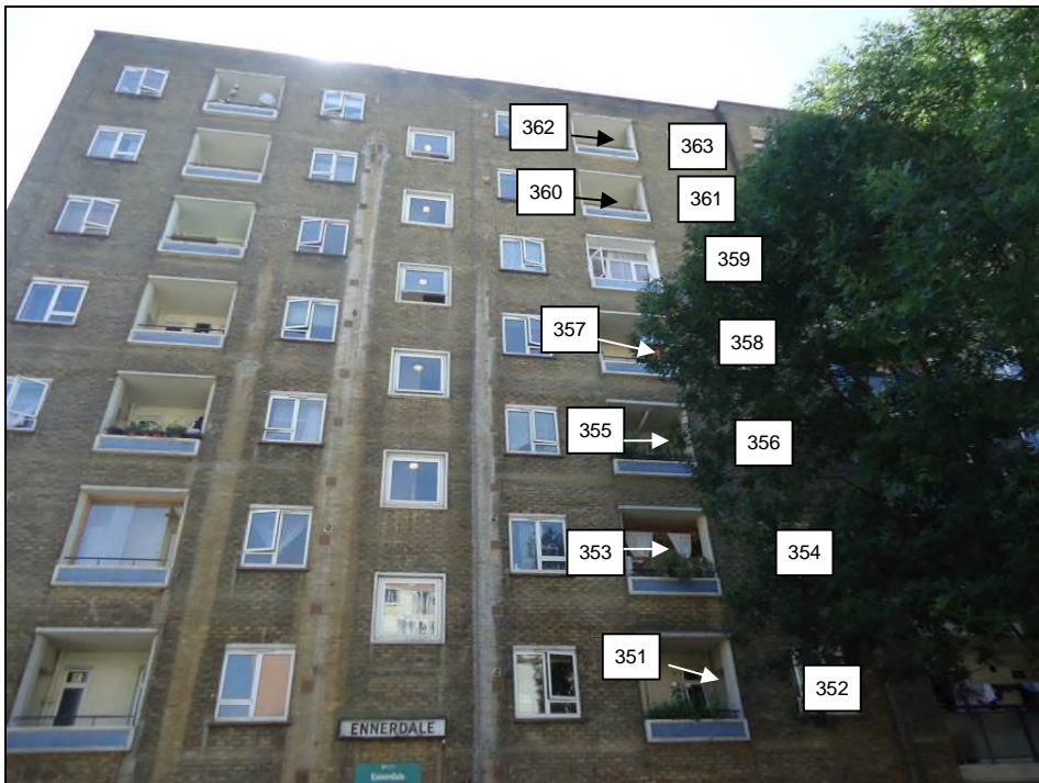
1 to 16 Ennerdale House
