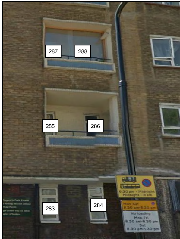
1 to 16 Ennerdale House
