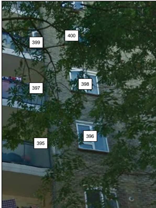
1 to 16 Ennerdale House
