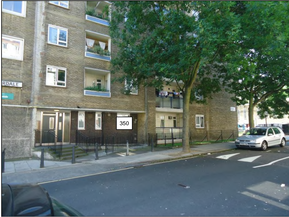
1 to 16 Ennerdale House
