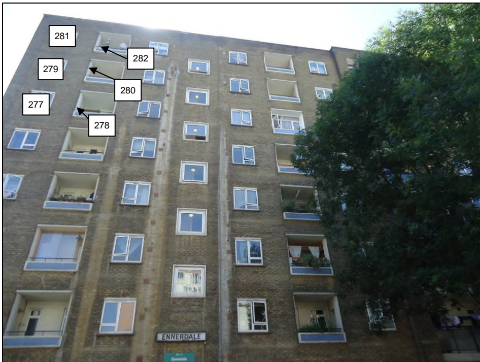
1 to 16 Ennerdale House
