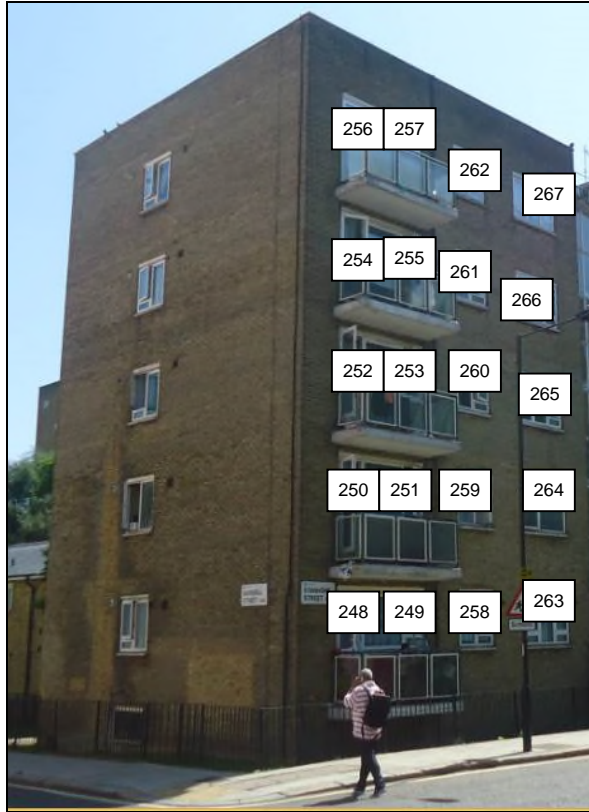
1 to 20 Stanhope Street
