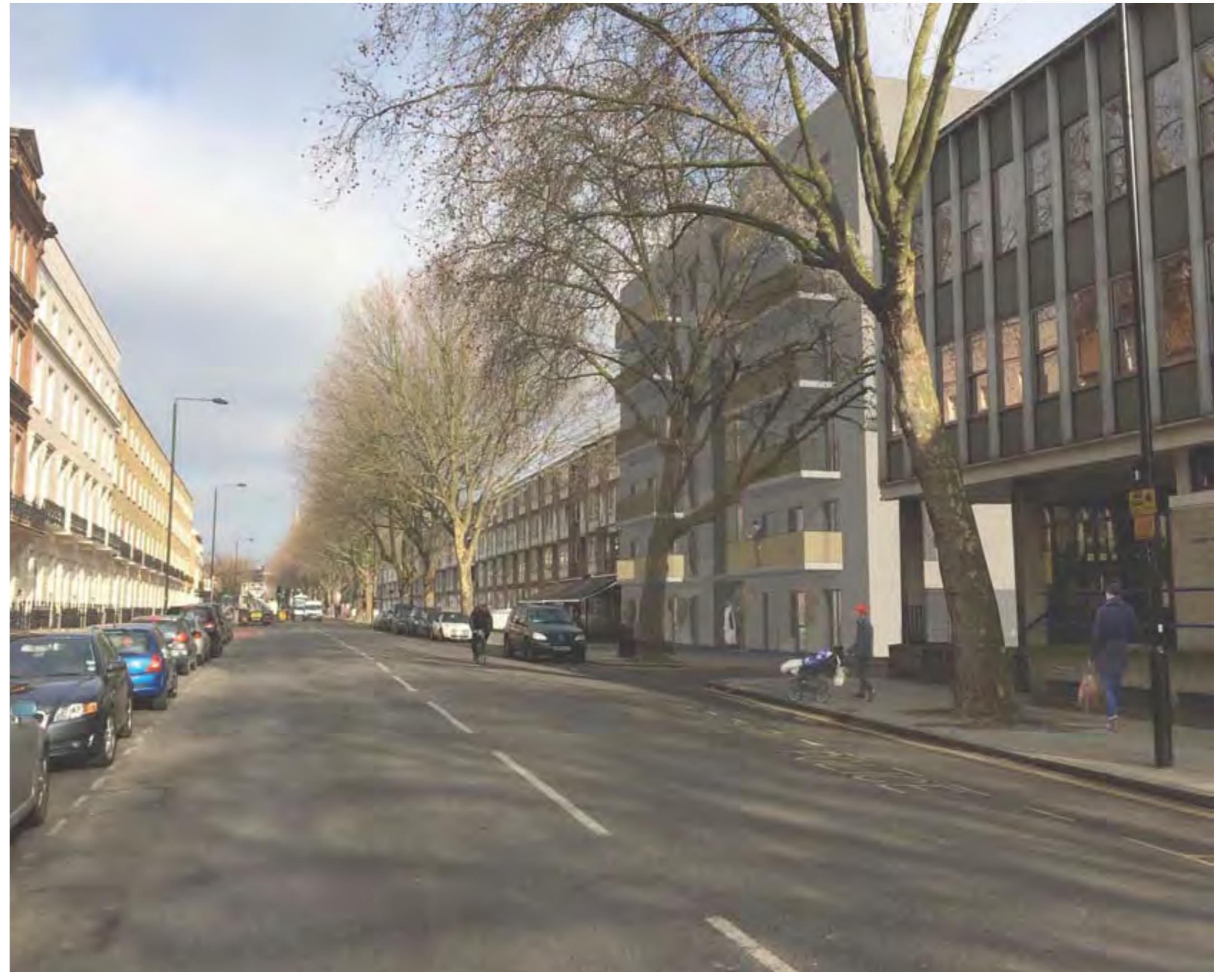
Street view of the proposal on the corner of Albany Street and Little Albany Street, creating a 'bookend' to Troutbeck, responding to the Nash terraces opposite
