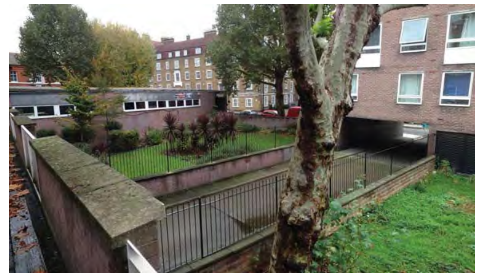
The existing courtyard space could be better designed, and we hope to improve this space as part of our proposals
