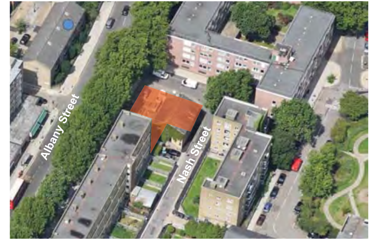
Aerial view of the existing site
