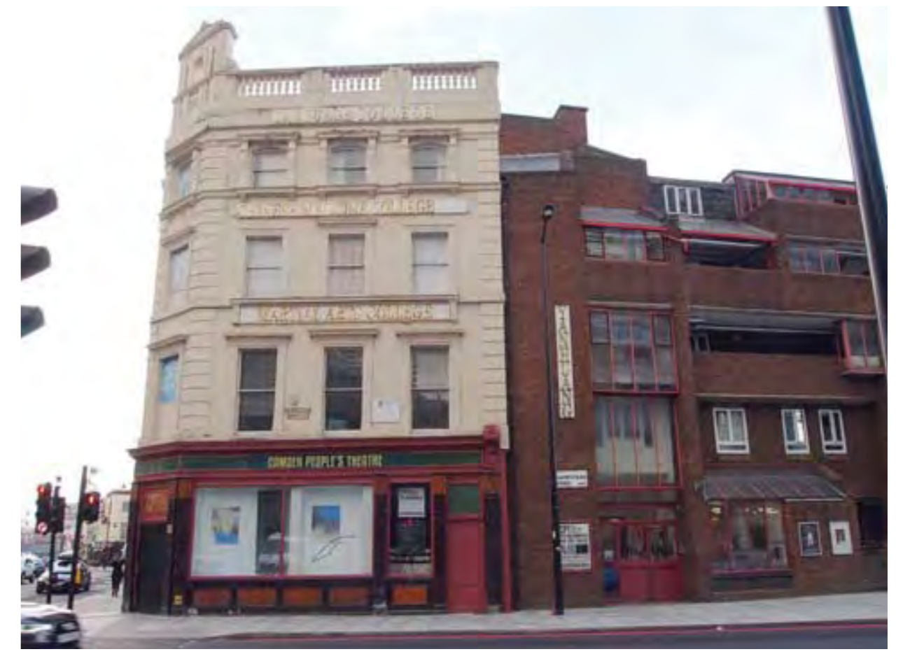
The existing CPT building has its access to the upper floors via the neighbouring building
