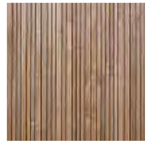
Timber cladding - Balcony
