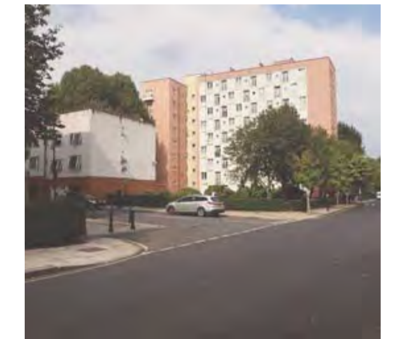
Current view to corner of site showing neighbouring flats and houses and open view into community garden.
