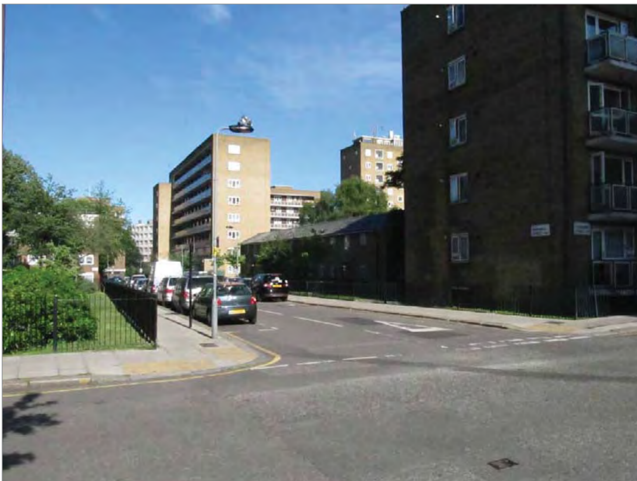
View of the existing Staveley block from Varndell Street
