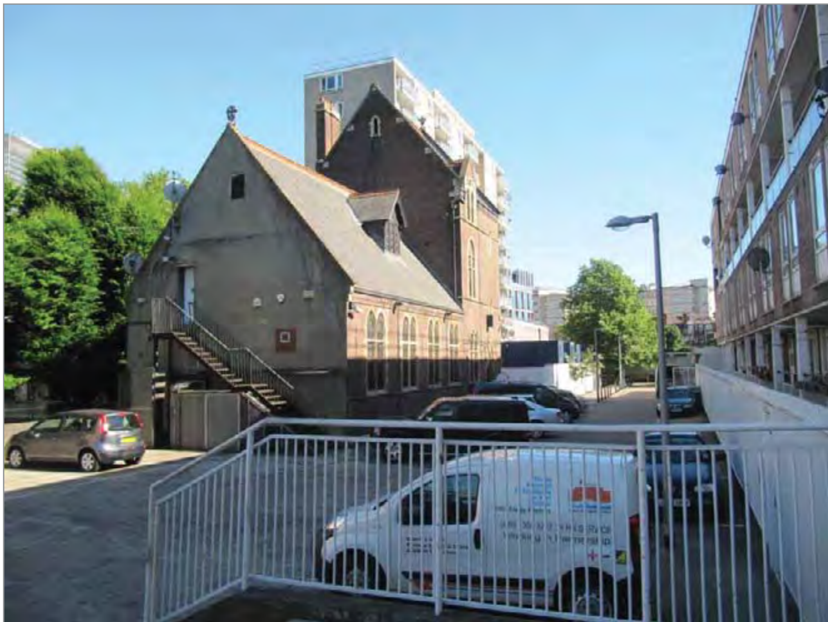
St Bede's is an attractive building within the estate, as seen from Troutbeck
