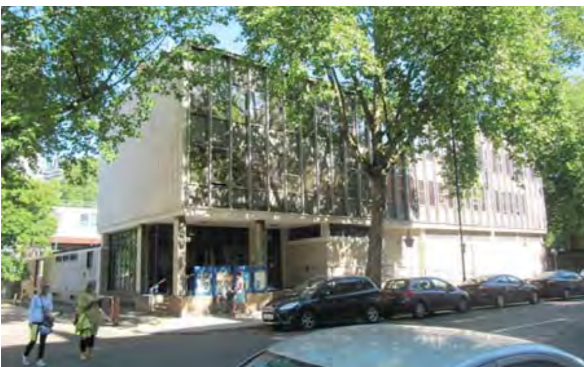
Existing: the former police station building
