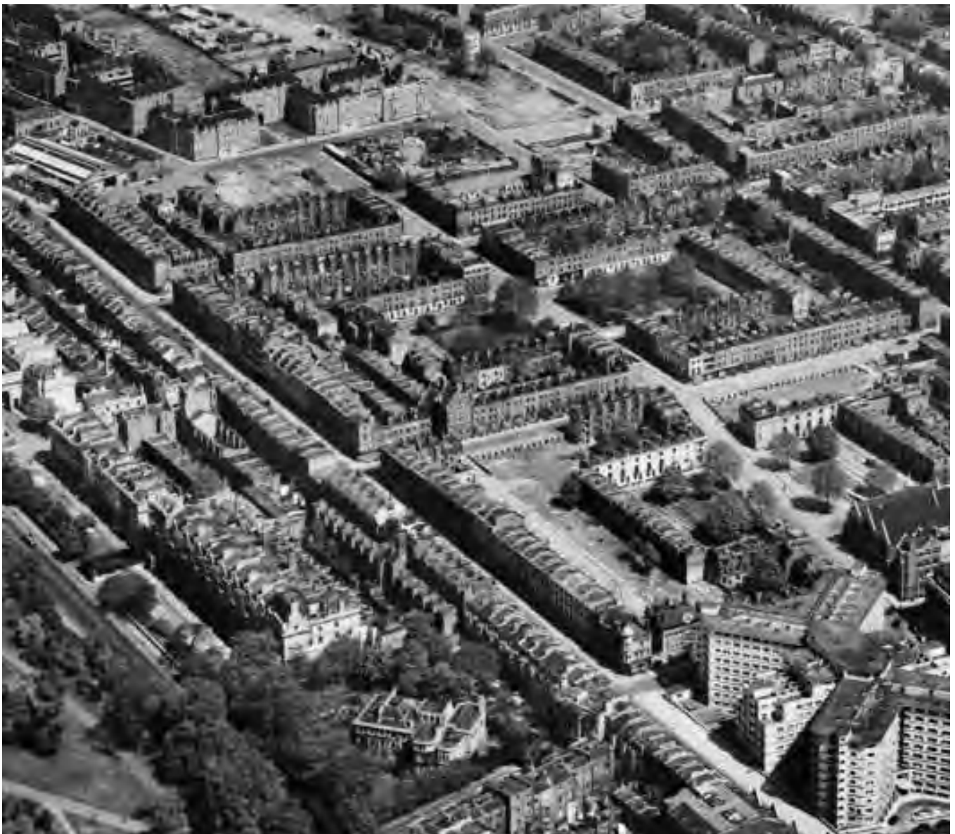
Figure 8: Aerial view looking north, 1948, showing relatively limited bomb damage. English Heritage, Aerofilms Archive.
