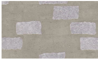
2. Granite setts within concrete path surface
