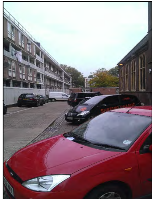
Photograph 4: Site 11 viewed from the east.
