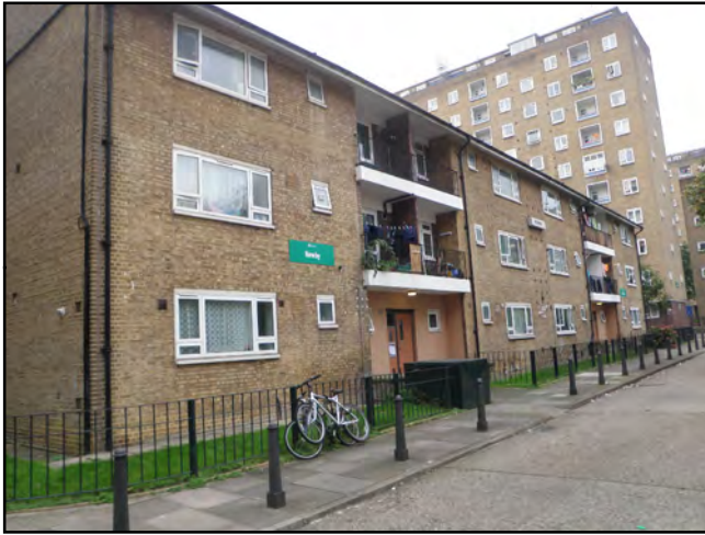
Photograph 5: Due to the presence of features including missing roof tiles, the Newby Overbuilds (Building 5) were assessed to have low overall potential to support roosting bats.
