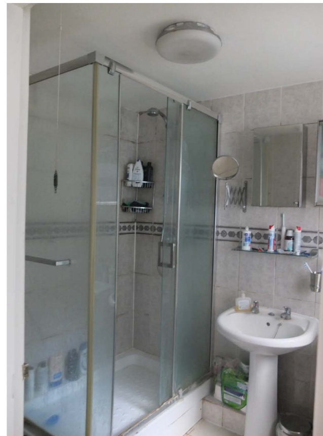
Existing basement shower room
