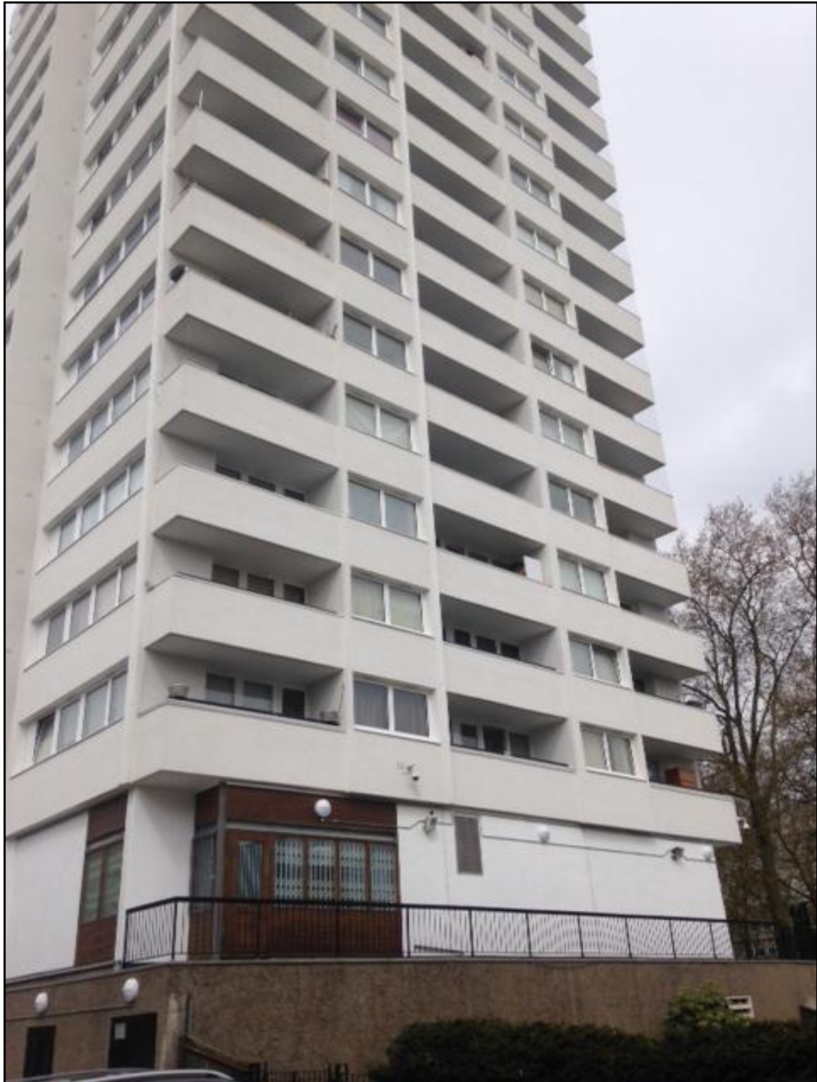
View towards subject property showing both balcony types
