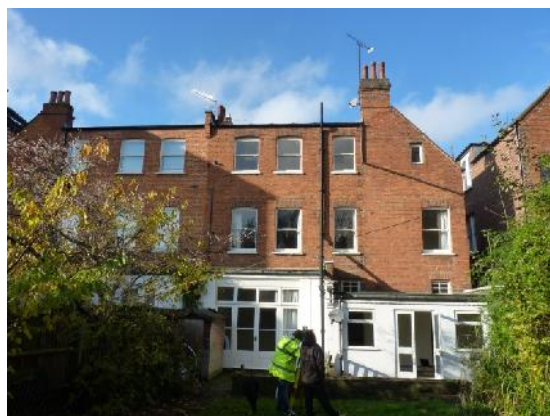
Views of context, entrance and rear of 4 Langland Gardens
