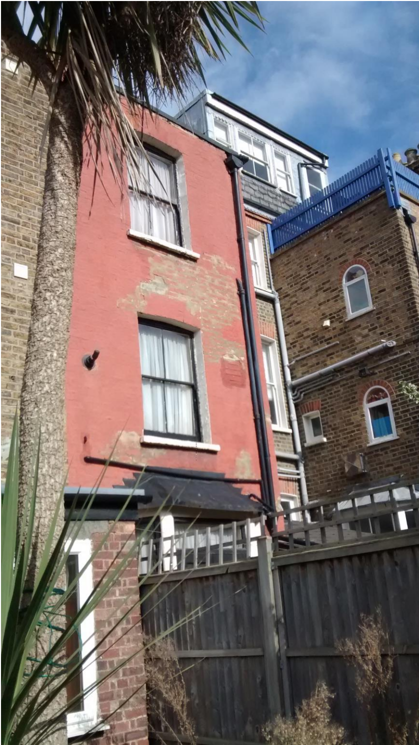
Figure 3 – Rear elevation of 17-15 Cotleigh Rd
